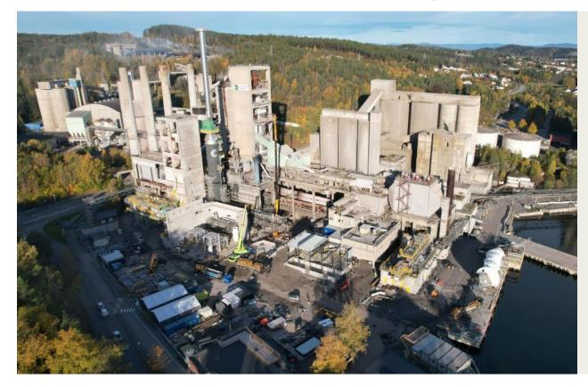
Demonstration plant 400.000 tons per year 55 tons per hour 50 % capture rate – limited by available waste heat 46 MW waste heat recovery
